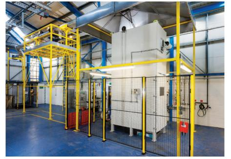
Side view of cable test chamber, hood and ducting
